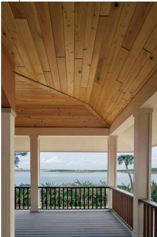
Native cypress distinctly panels the ceiling of the wraparound porch, complimenting the views of the lake.
