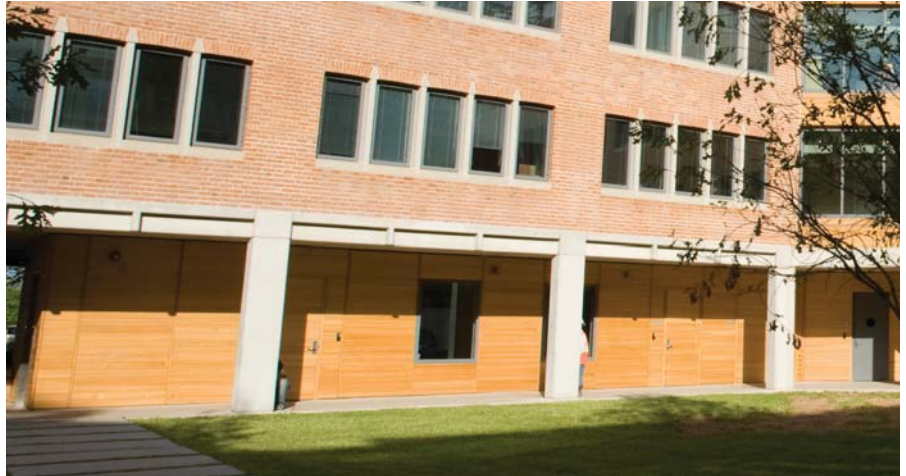
NEW RESIDENTIAL COMPLEX at Rice University, Houston, Tx., where vertical-grain cypress wraps the first-floor exterior, extends as paneling into an interior entry, and then up a stairway to the second floor. Window trim is also cypress. (Photo by Rice University)
