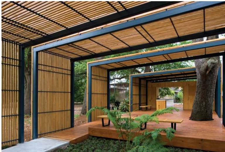
HURRICANE-DOWNED cypress from New Orleans' Botanical Park was used to construct a modular pavilion that was built for garden volunteers, but is also used for meetings, seminars, and parties. (Photo by Mike McKay, Lexington, Ky.)
