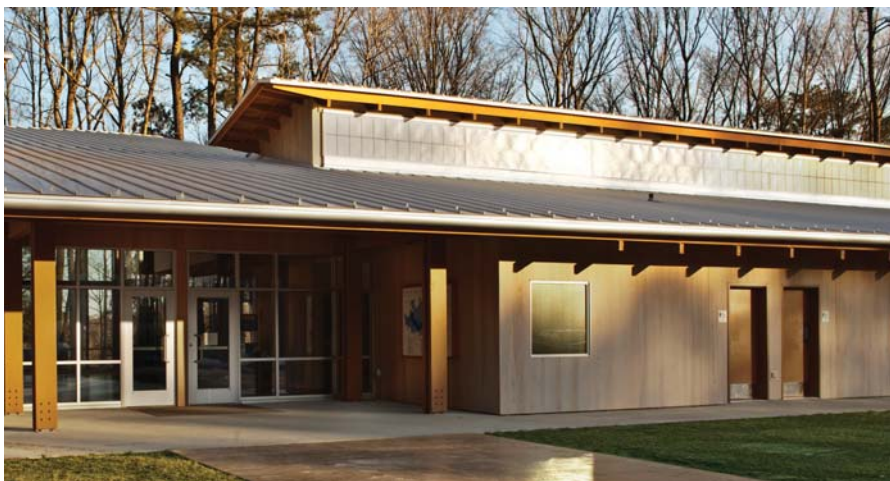
CYPRESS reclaimed from the nearby Great Dismal Swamp National Wildlife Refuge was milled into siding for the Merchant Millpond Visitor Center, Gatesville, N.C. (Photo by Richard Leo Johnson, Atlantic Archives Inc., Savannah, Ga.)
