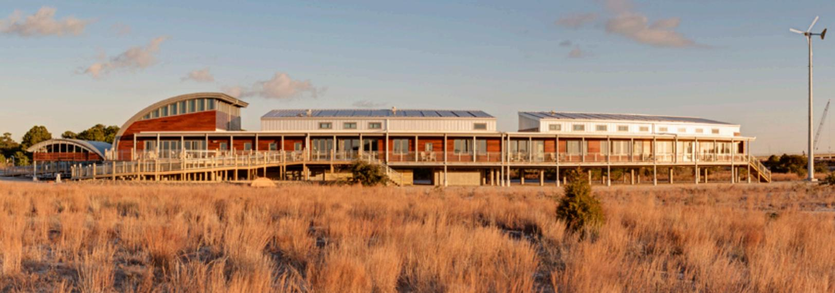
“Cypress contains a preservative oil called *cypressene*, which makes the wood naturally resistant to rot, decay, and insects,” Mella explained. “Given its natural durability, we clad the exterior walls in 7,800 square feet of shiplap cypress, finished with a stain to provide protection from ultraviolet light and to give the wood a rich, warm tone.
