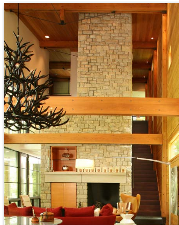
Cypress flitch beams and trusses were used to add architectural support and detail.
