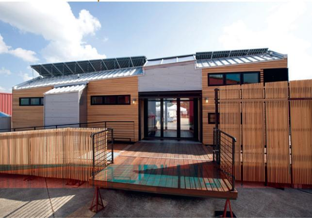
Above: The exterior of BeauSoleil features an innovative cypress rain screen that helps minimize heat gain.
