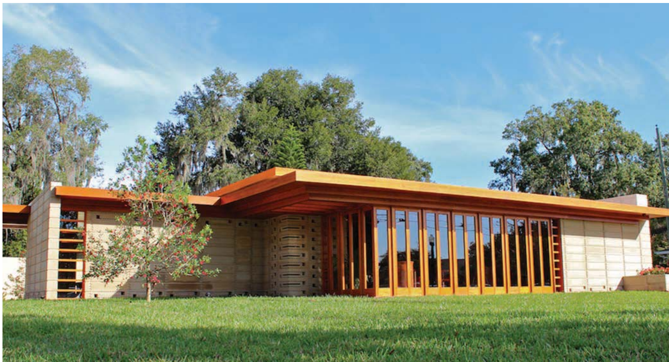
USONIAN HOUSE , newly constructed at Florida Southern College, Lakeland, Fl., showcases Frank Lloyd Wright's affinity for cypress and other locally sourced materials, such as handmade bricks and other natural materials. (Photos by Michael Maguire, www.buildingtheusonianhouse.com )
