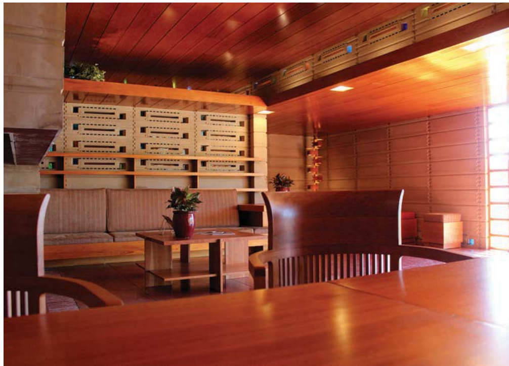
CYPRESS is heavily featured in the interiors, used anywhere a finished wood product was required, including all interior ceilings, plank walls, built-in cabinets, light fixtures, and furniture.
